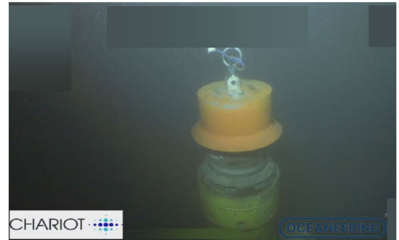
Installing Temporary Abandonment Caps
